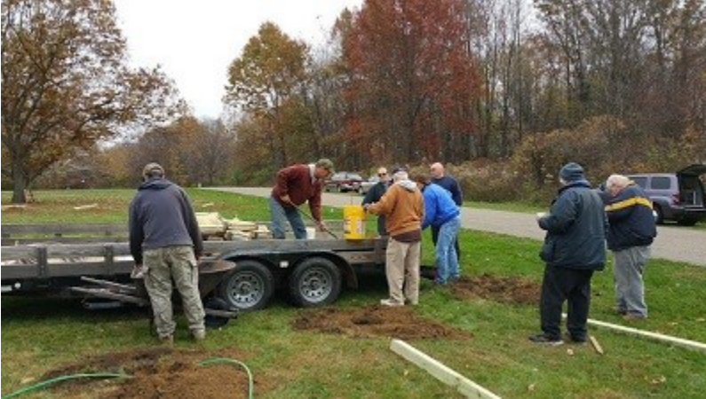
ACA members and friends starting the first stages of building the observatory fence to block car lights during observing sessions. Image by ACA member Glenn Cameron.
